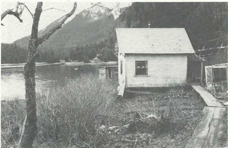
Boardwalks and trails are the primary means of overground access in Kupreanof; however, most travel in this community is by skiff.
